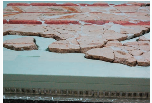
Fig. 5. Detail of the new wall painting support frame, consisting of a rigid panel and two intermediate layers that surround the piece.
