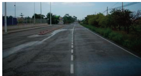
Figure 4. The modern Camí de Vizcarra. One of the preserved decumani of a centuriation.
